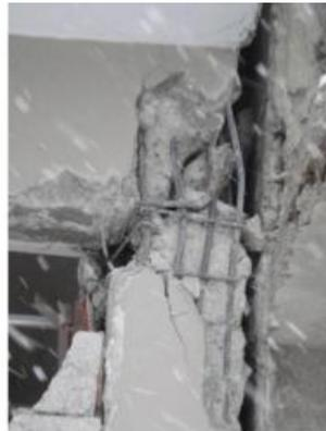
a. Beam-column joint without proper design. Van earthquake in Turkey, 2011 [5].
