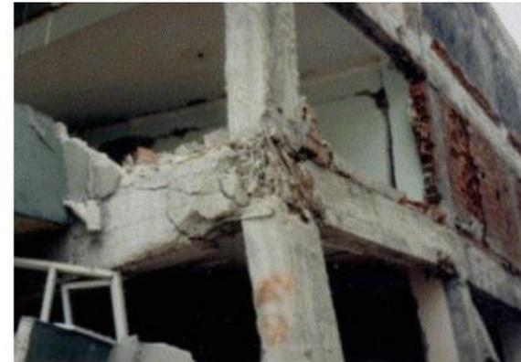
b. Insufficient lateral ties at the joint [11].
