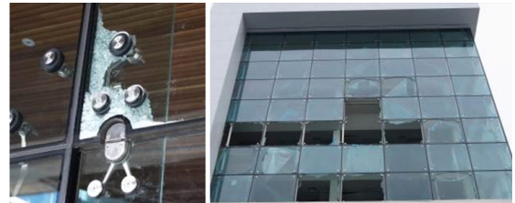
b. 2011 Christchurch earthquake (spider glazing system)
