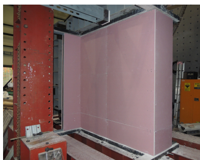
(a) Installation of test specimens
